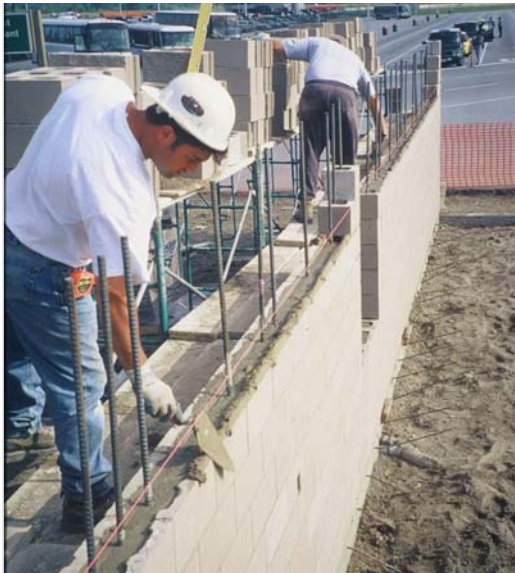
Figure 3. Confined masonry construction in Indonesia (top) 4 and reinforced masonry construction in Canada (bottom) 5
